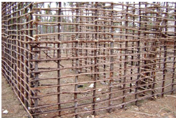
Figure 1. Traditional house under construction composed virtually of mangrove poles. (© J. Lang'at).
