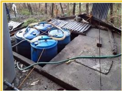
Novel Low-Cost Plastic Drum Biogas Digester designed by Dr. Antonio J. Barroga of CLSU [30]
