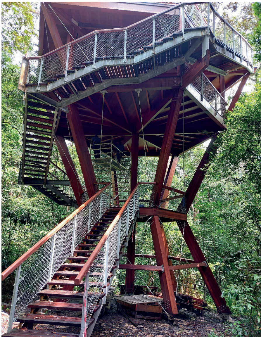
Treetop classroom made of padouk, Raponda Walker Arboretum, Cap Estérias, Gabon Ecwood production (© Emmanuel Groutel, WALE)
