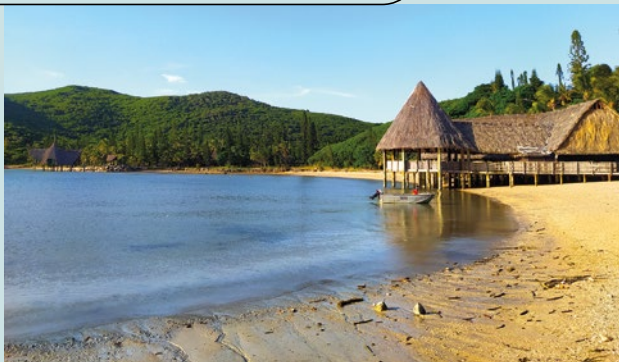
Photo 1. Covered dock, made with wooden poles in radiata pine ( Pinus insignis ) treated with CCA (Chromated Copper Arsenate), Nouméa, New Caledonia, France. Photo K. Candelier.
