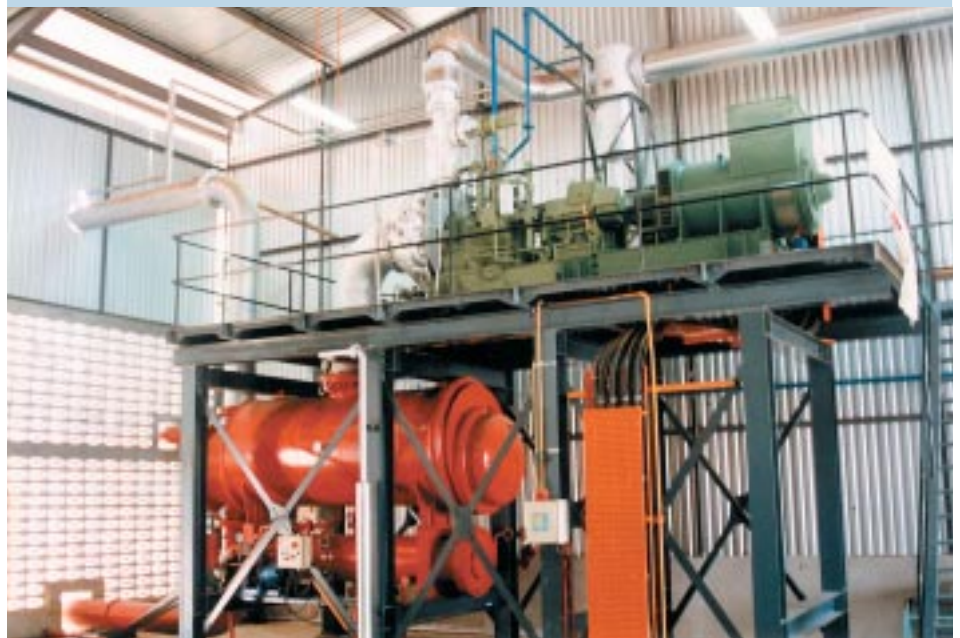
Turbine à condensation Nadrowski (900 kW). Nadrowski condensing turbine (900 kW). Photo P. Girard.
