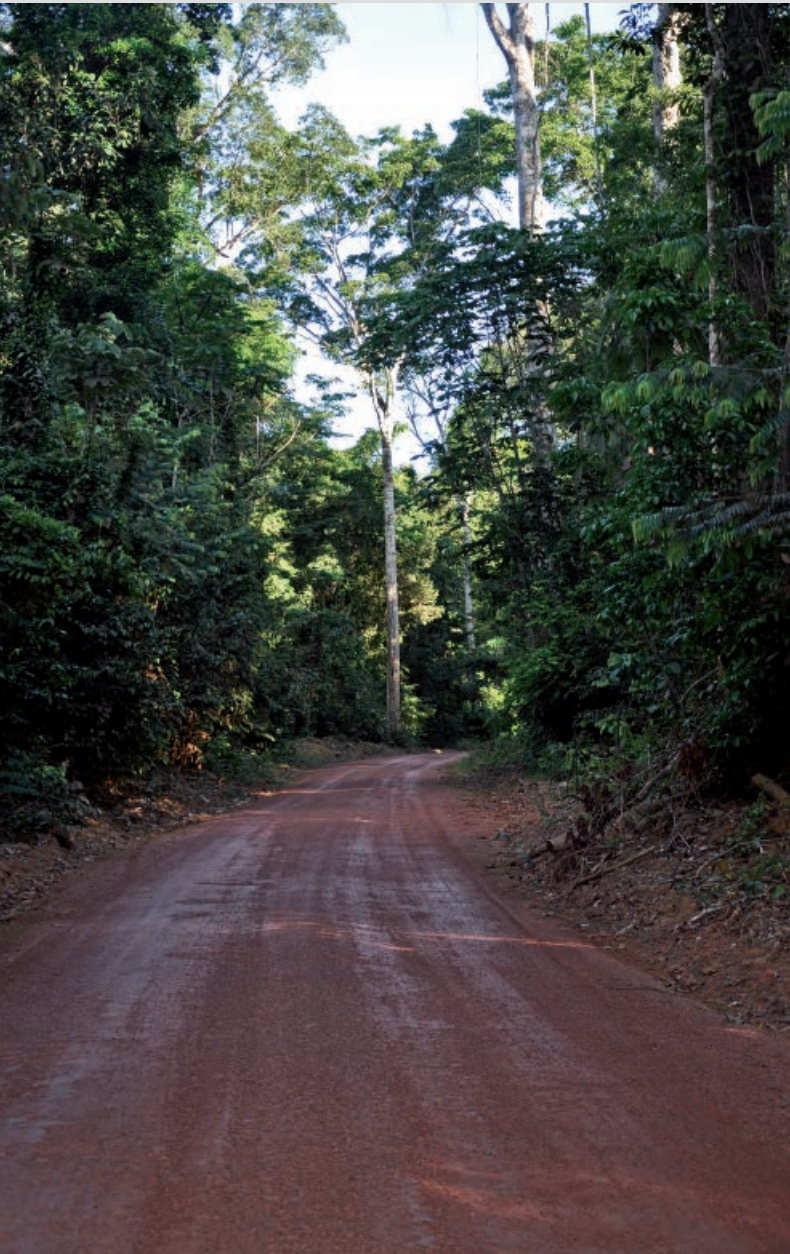
Forest road at Cikel in responding to the RIL techniques requirements (limited width of the road). Photograph P. Sist.
