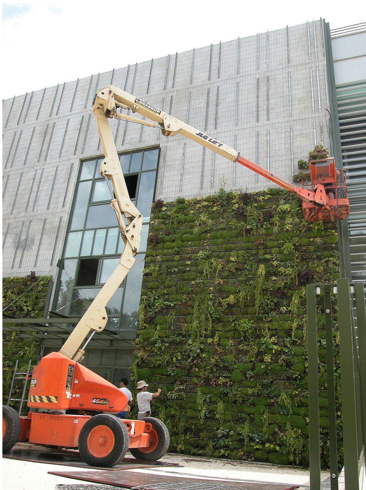
Construction of a modular plant wall (entrance frontage of the tropical greenhouse of the Montpellier's Zoo)
