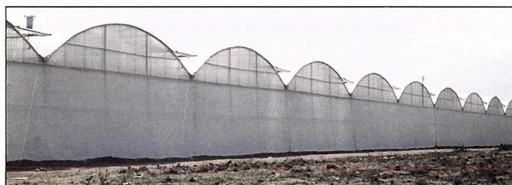
Double ridge continuous vents
