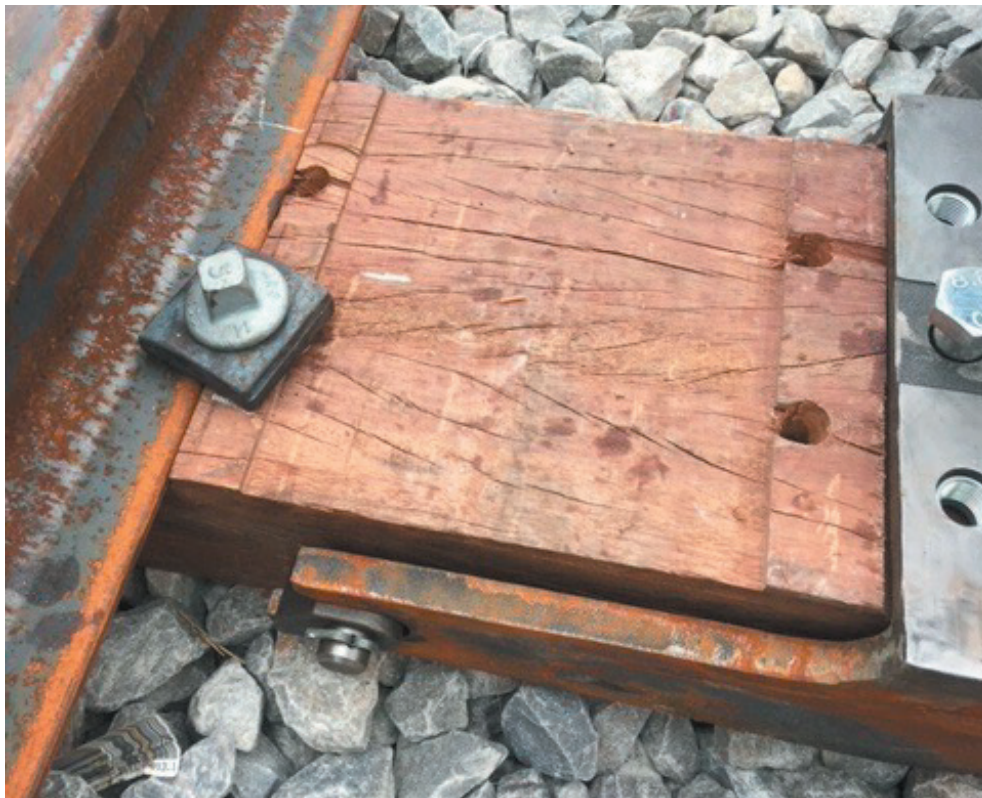
Detail of the assembly of an Azobe part (rail/tyre) for metro line no. 6 in Paris (photo: Rail Europe)
