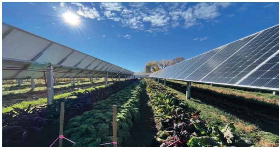
Fig. 1.22. Illustration of co-location of solar PV panels and agricultural land with cropping. Reproduced with permission
