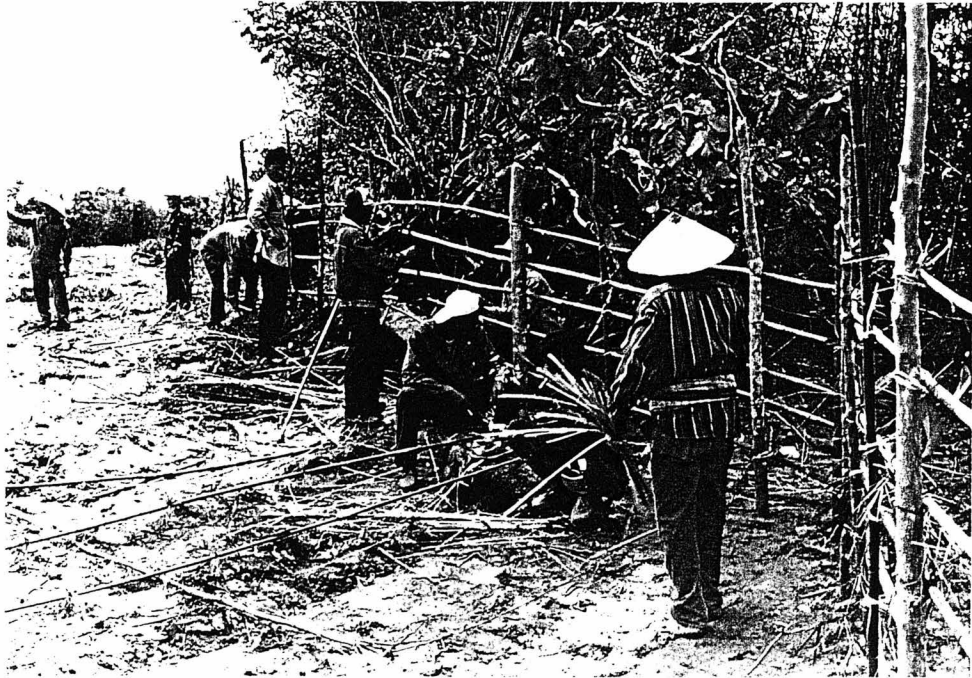
Photo 5. One of the extension activities was a working field day for the Lao Youth Organisation assisting with fence construction and planting hole digging at the Na Kaha PBP in Vientiane Prefecture.
