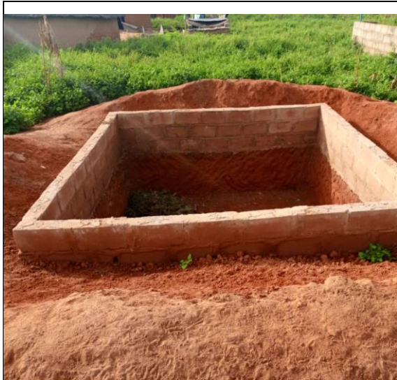
On-going construction of manure pit in Dafinso
