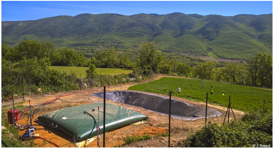
Figure 6.1. Experimental site for water reuse, Saint-Martin-de-Castillon (Vaucluse)
