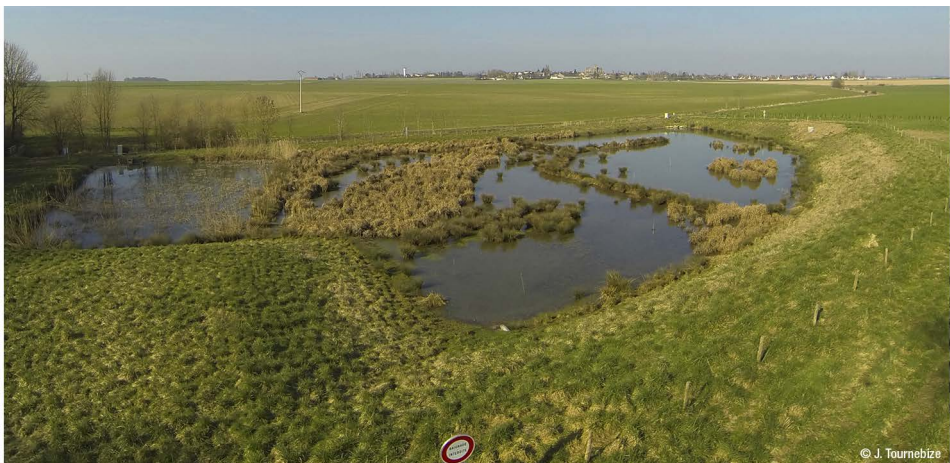
Figure 6.3. Artificial wetland buffer zone (AWBZ) in a crop farming context, Seine-et-Marne
